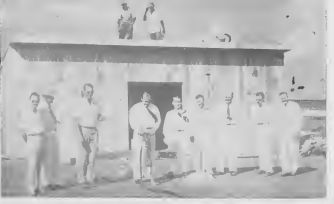
As Company officials and construction supervisors look on, J. J. P. Oubler officially breaks ground for the addition to the Main Office Building that will house the IBM equipment. From left to right are: Mr. Lester, TSD coordinator, George Brinkman and Hugo Swettenham, vice-president and general representative respectively of the IBM (International Business Machines) Company, Mr. Oubler, head of the Tabulating and Statistical Division which handles IBM equipment, J. H. Nunes, technical superintendent, O. Minguo, acting general manager, C. A. Currier, chief electrician, E. L. Ward, TSD coordinator, and T. C. Brown, comptroller and head of the Accounting Department.
